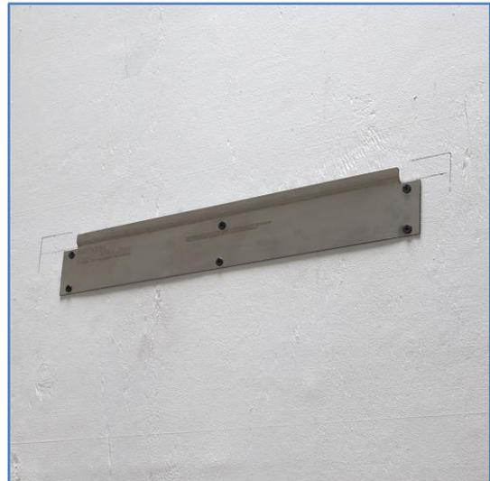
**Figure 7:** Mounting bracket installed on wall (fasten center holes if wall studs are unavailable)
