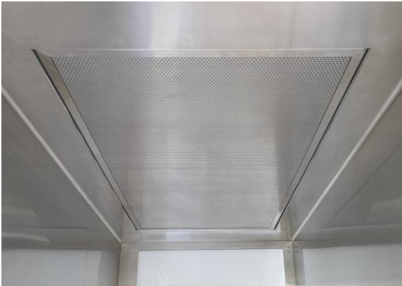
Figure 12: A stainless steel screen hides the HEPA filter
