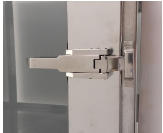
Figure 8: Properly aligned LiftLatch
