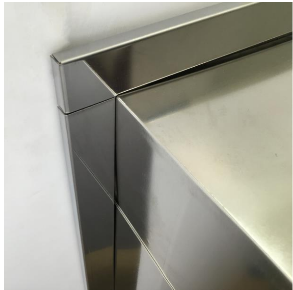
Figure 7: Snap the bracket covers back into place to hide the lag bolts and other hardware
