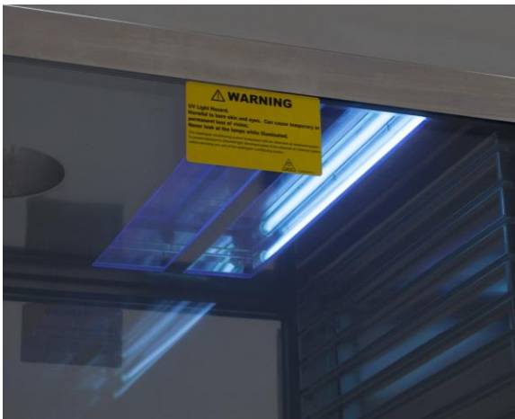
Figure 10: Recessed UV-C light
